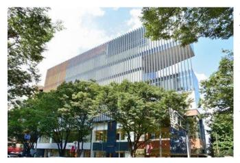
**One Omotesando** (Kengo Kuma / 2003.09) mullion contributes The to energy conservation by shielding the interior from direct sunlight and mitigates the greenhouse effect by fixing carbon dioxide production. Although Japan's Building Standard Law prohibits the use of wood on the exterior walls of buildings in large urban areas we were able to obtain special permission by installing a drencher on the outside wall.
